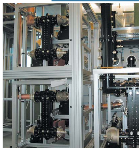
8-way transmitter combiner for the television tower Berlin-Alexanderplatz
